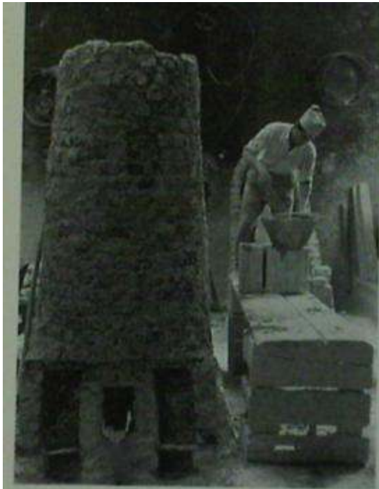
2.9 The completed baking oven, with two channels for fuel and one for wax escaping from the molds. Courtesy of Alison Frantz.
