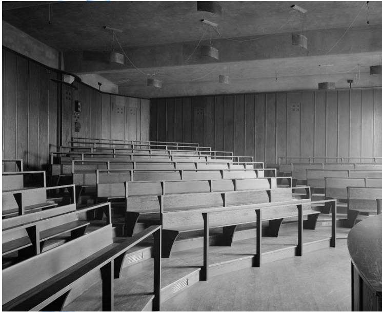
Lecture theatre, photograph by Bedford Lemere, 1910
