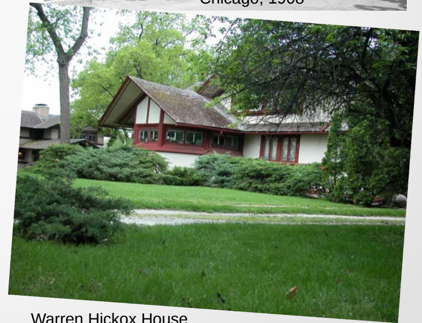
Warren Hickox House (1900), Kankakee, Illinois,
