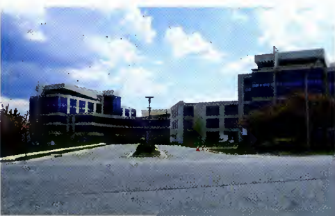
Business park, near Heathrow airport, London
